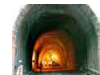
Main Access Tunnel - under construction Punatsangchu-I.H.E. Project, Bhutan
