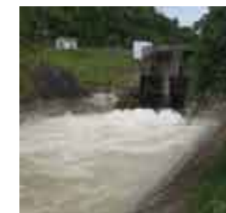
Nam Song Hydro Power Project, Laos PDR
